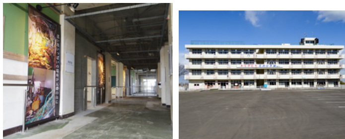
Sendai Arahama Elementary School
