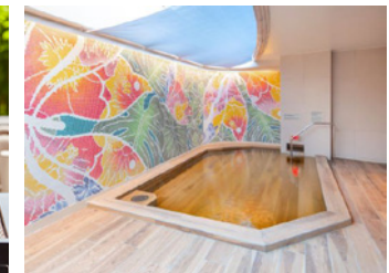
Local natural gas heats the spa water in this hotel
